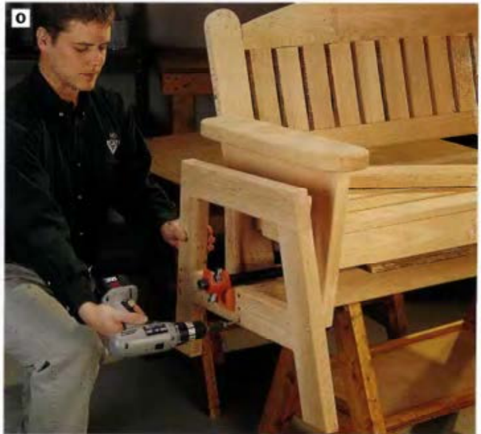
PHOTO O: Install stretchers between the end assemblies of the glider stand with 2½-in. countersunk flathead wood screws. Clamp the stand's ends to hold them stationary as you fasten the stretchers in place.
