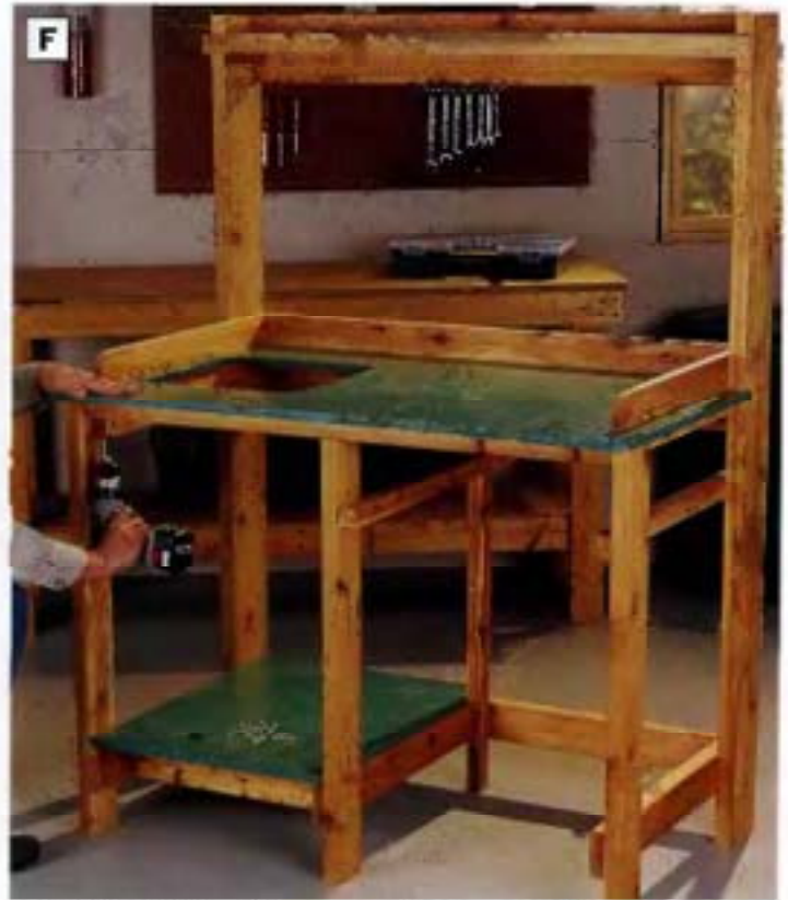
PHOTO F: Install the back splash and side splash pieces on the countertop, then fasten the countertop to the bench framework by driving screws through the stretchers from below and into the countertop.
