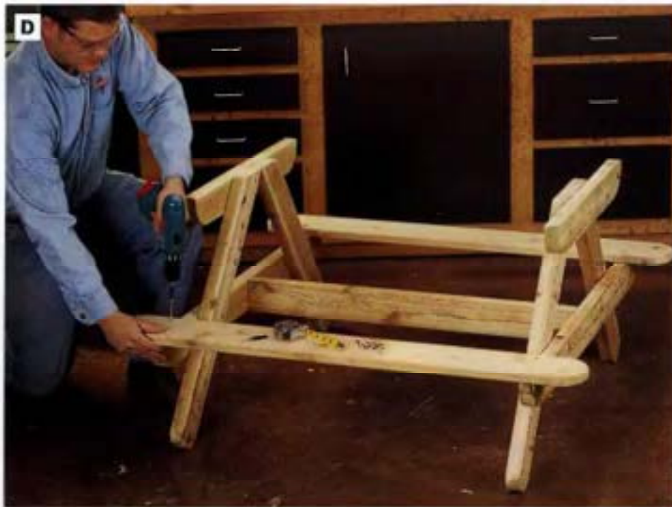
PHOTO D: Set the frame upright on the floor to secure the seats into position. The ends of the seats should overhang the seat stringers by about 4½ in. Make the outside edges of the seats overhang the ends of the seat stringers by 1 in.
