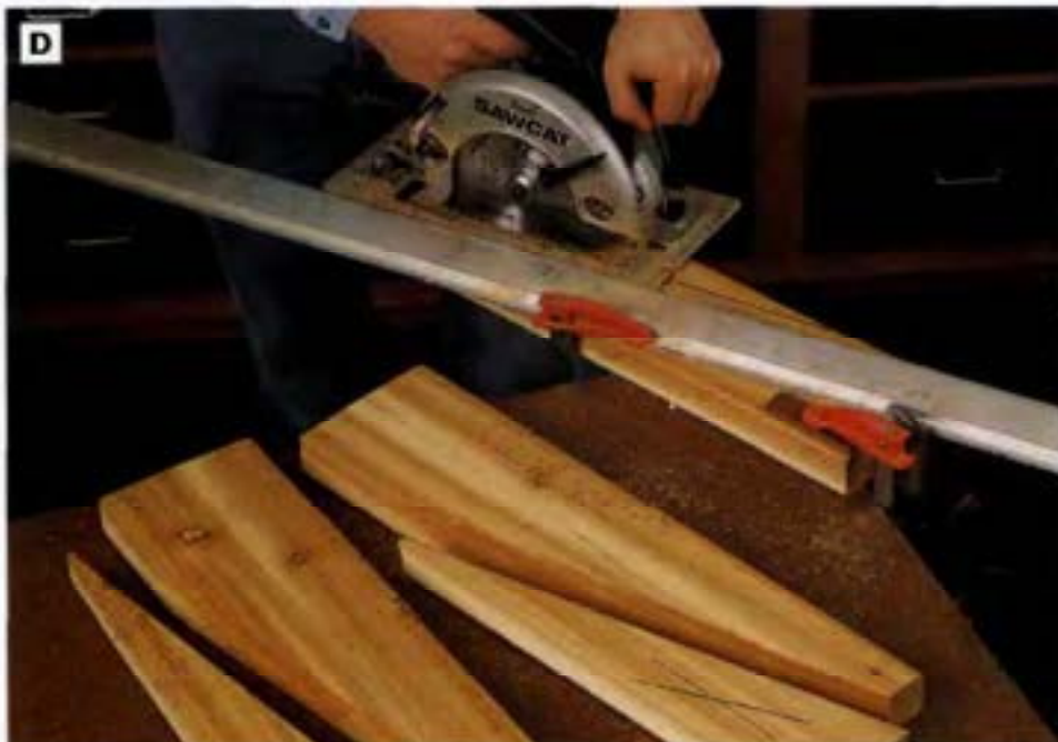
PHOTO D: Cut the back supports to shape with your saw guided against a straightedge.
