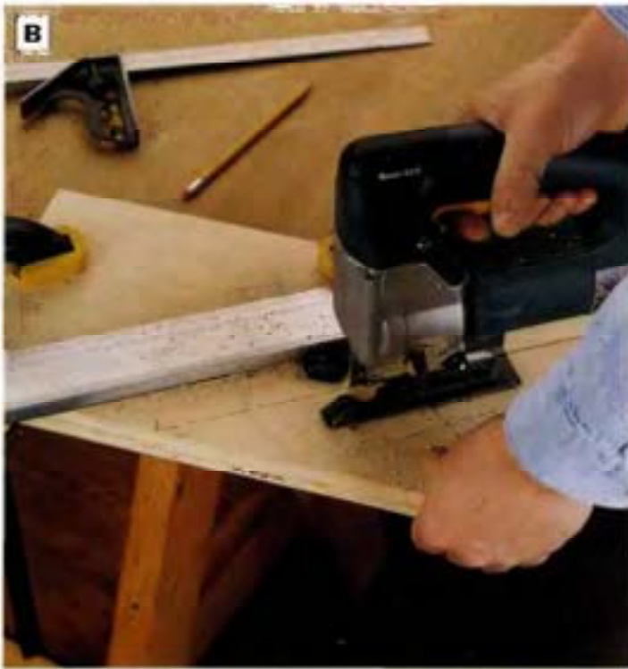
PHOTO B: Lay out and cut the side panels to shape with a jig saw guided by a clamped straightedge.
