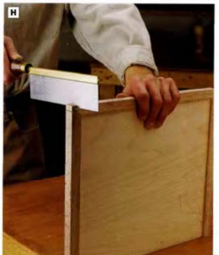
PHOTO H: Cut \frac{3}{8} × \frac{3}{8} -in. notches in the outside corners of the tray to allow it to fit around the inside corners of the legs. Use a small, fine-tooth saw like the dovetail saw shown above. Make sure to keep the tray plumb as you cut.
