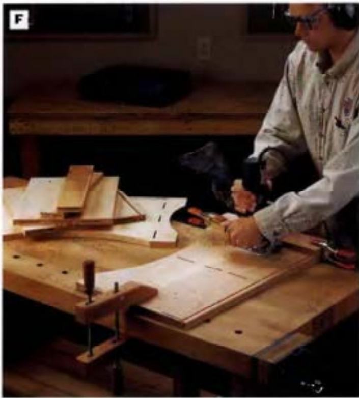
PHOTO F: Cut biscuit slots in the sides and in the ends of the bottom, top stretchers, and shelf for assembling the carcass. Clamp a plywood straightedge to the side panels to help align the base of the biscuit joiner when cutting biscuit slots in the side panels.
