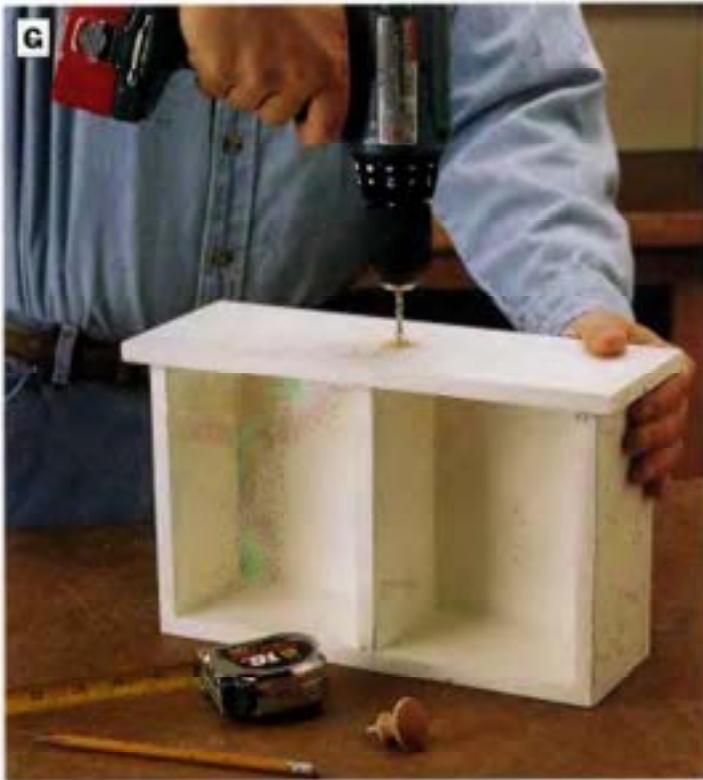
PHOTO G: Drill a pilot hole at the center of the drawer front for a threaded drawer pull. Install the pull.
