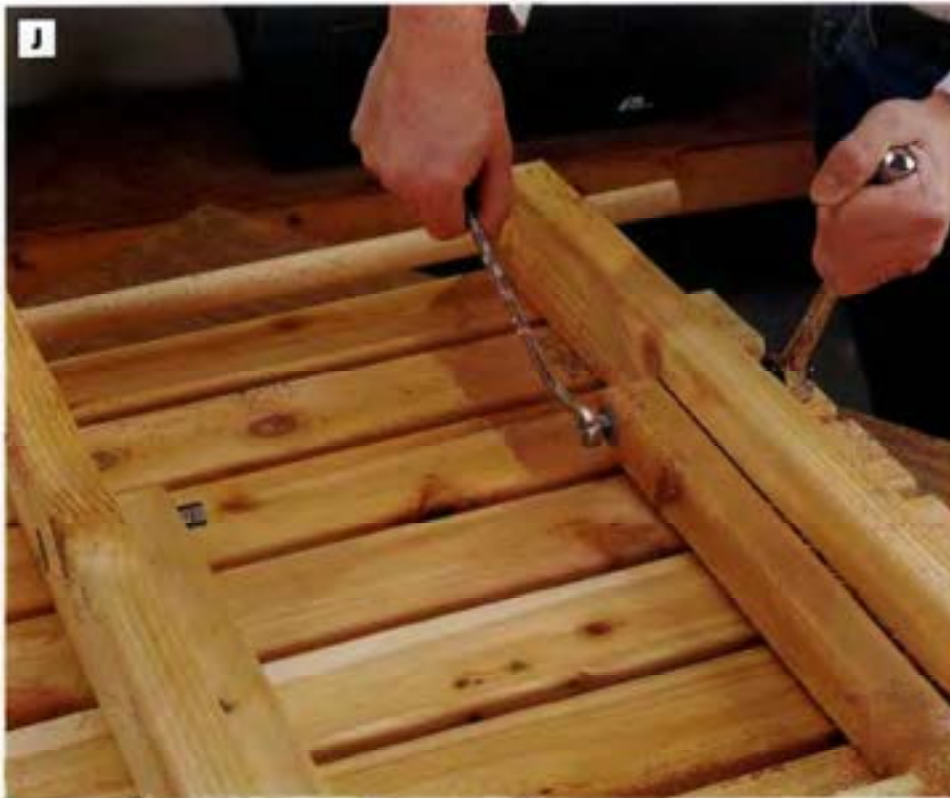
PHOTO J: Install the adjustment brace to the back rest with bolts, washers and nuts. Place a washer on either side of each adjustment brace. Thread two nuts on each bolt and tighten the nuts against one another to lock them together, yet allow the adjustment brace to swing freely.
