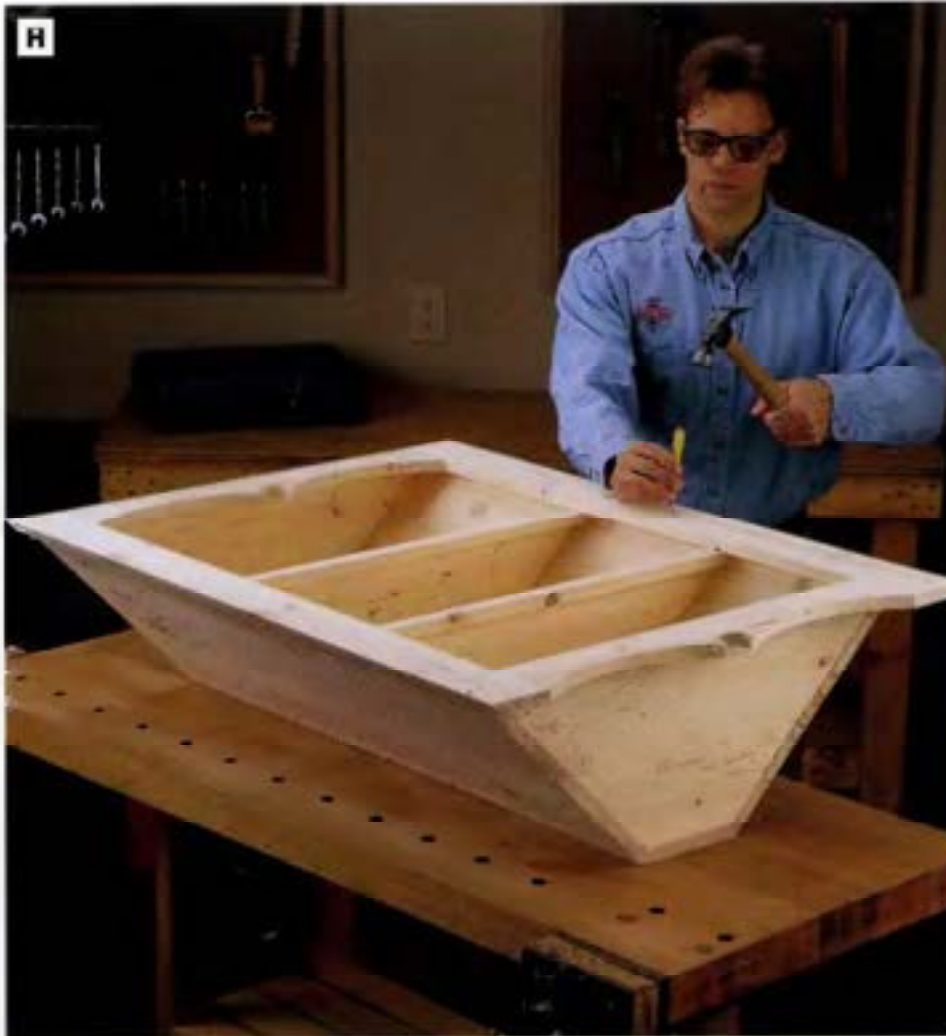
PHOTO H: Attach the face frame to the cupboard carcass with glue and 4d finish nails. Drive the nailheads below the face frame surface with a nailset.
