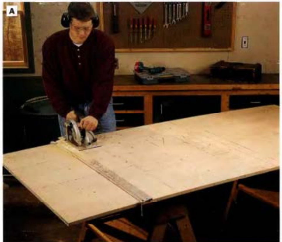
PHOTO A: Draw a cutting diagram on the plywood sheet to lay out the project parts. Mark each part with a letter that corresponds to the Cutting List on page 272 to help identify them. Clamp a straightedge in place to guide the saw as you cut the parts to size.
