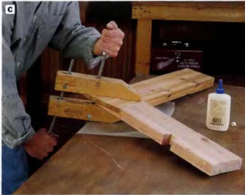
PHOTO C: Glue and clamp the half-laps of the seat supports and the back supports together to create L-shaped blanks for the three support structures. Use weatherproof glue.
