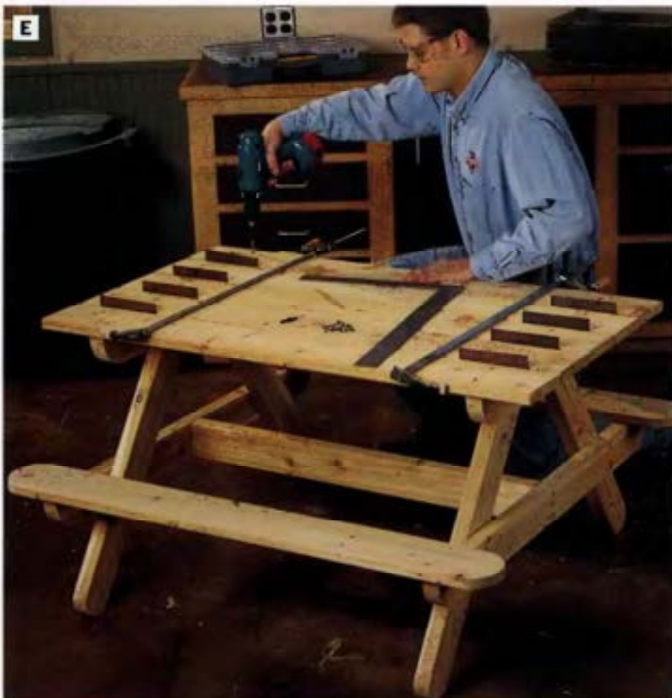
PHOTO E: After setting the slats into position on the top stretchers and marking alignment lines for screw holes, insert spacers between the slats—we used ¼-in.-thick hardboard. Clamp the top slats together to keep them aligned, and fasten them to the top stringers with countersunk 2-in. deck screws.
