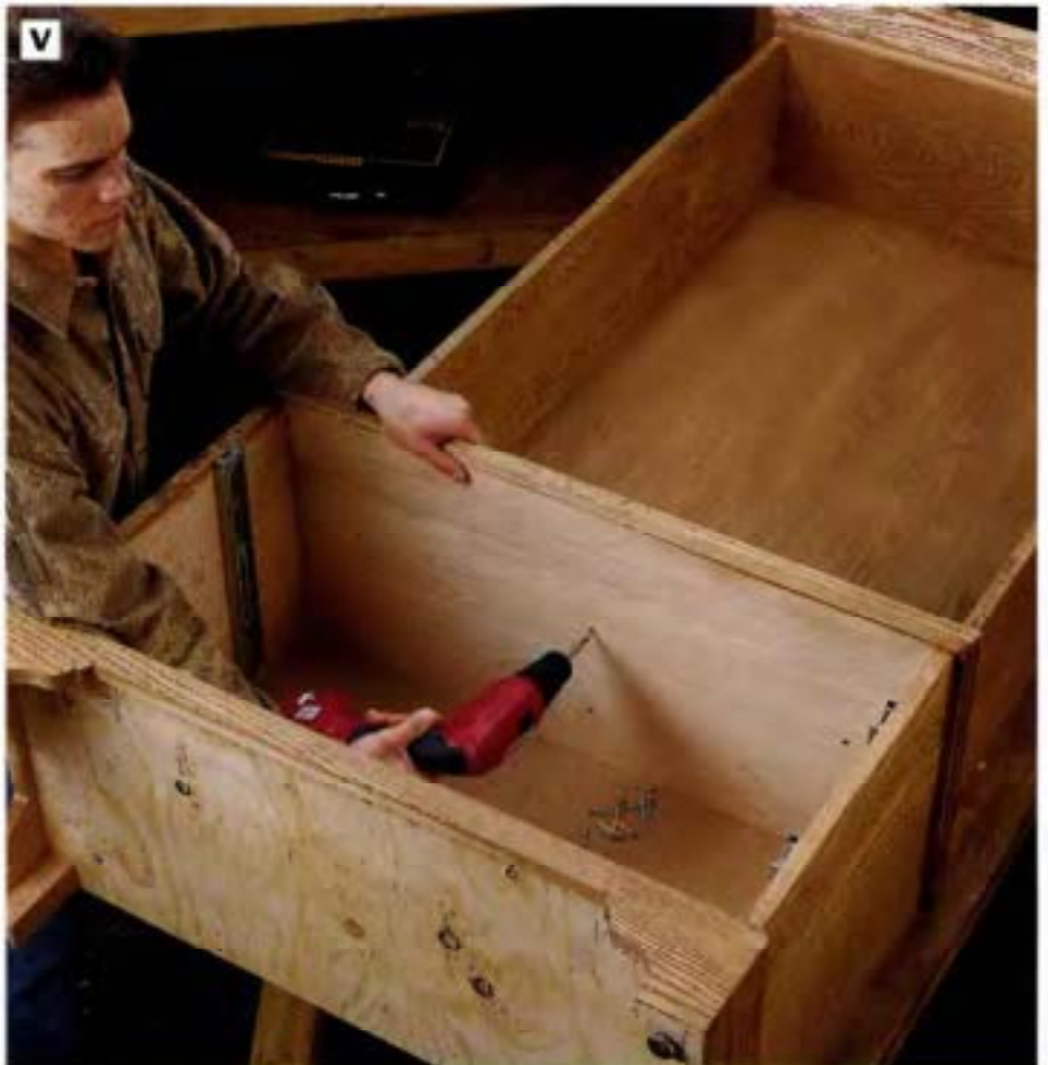
PHOTO V: Screw the upper and lower cabinets together. Lay the cabinets down so their backs are flush. Center the upper cabinet on the lower cabinet, side to side, and hold them tightly together. Drill countersink holes for the screws (a tapered countersink hole will allow the screws to draw the parts together tightly).
