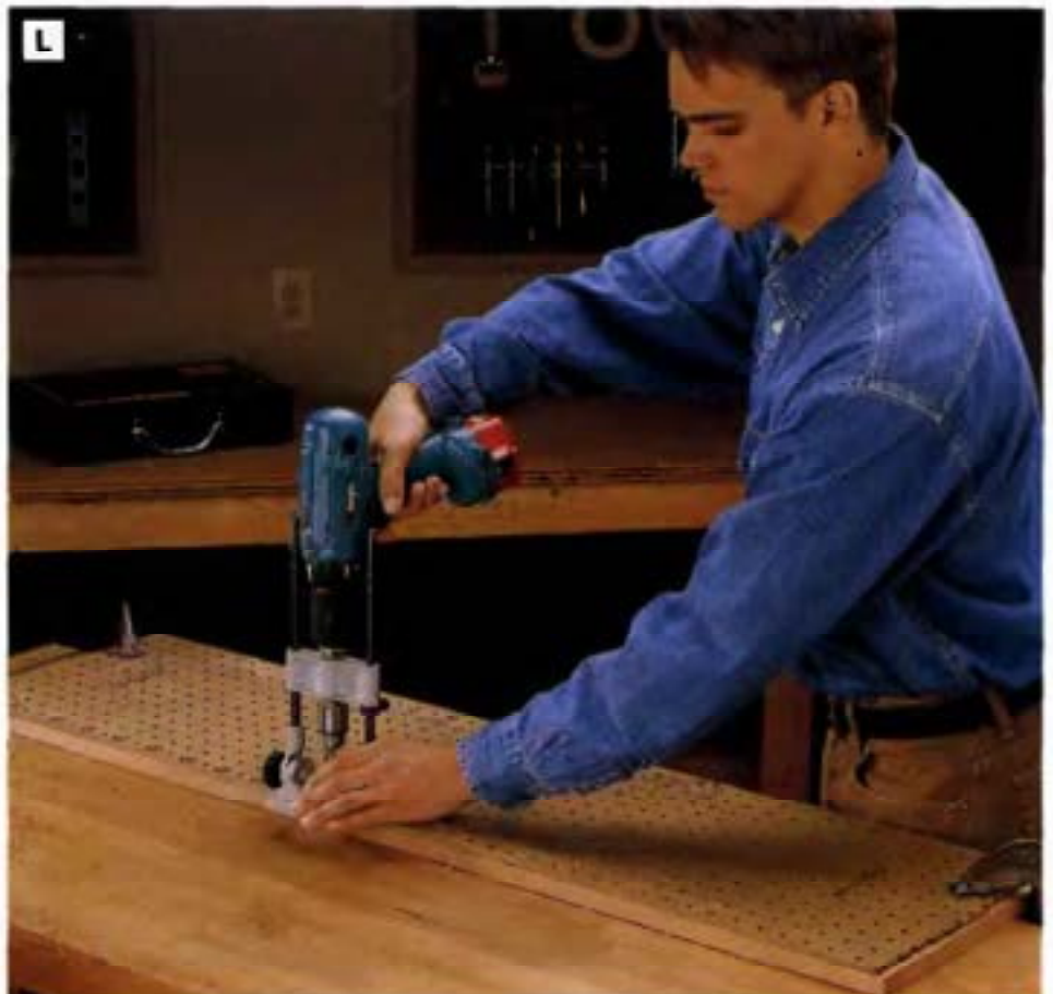
PHOTO L: Drill shelf pin holes in the side frame stiles using a piece of perforated hardboard as a template and a drill guide to ensure perpendicular holes.
