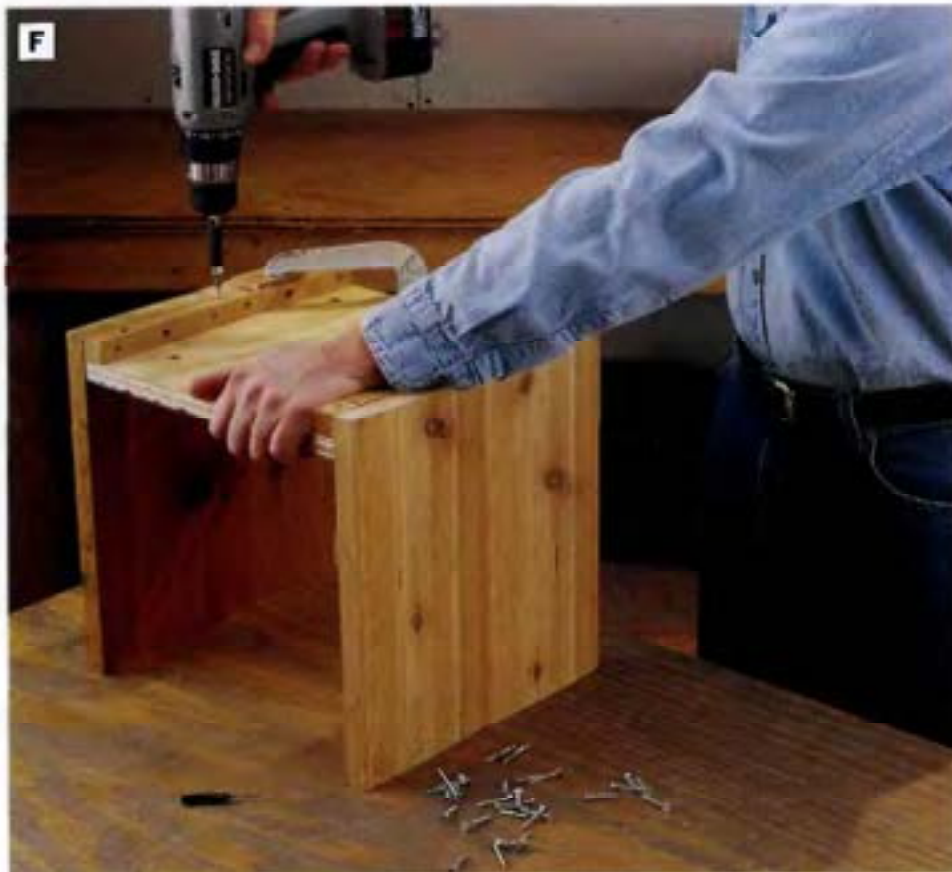
PHOTO F: Cut the bottom piece to size, drill five weep holes through the bottom for drainage, and fasten it to the cleats on the end pieces with countersunk screws. Attach the bottom so it will rest on the cleats when the planter is finished.
