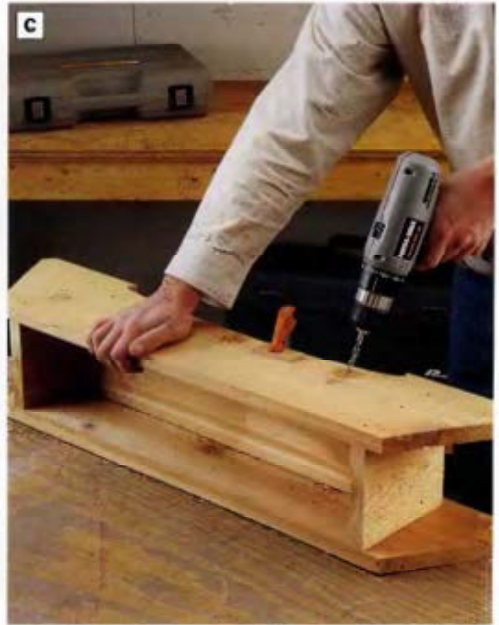
PHOTO C: Fasten the planter sides to the ends and bottom with nails, then drill three angled \frac{1}{4} -in.-dia. weep holes through the side where the bottom of the planter slopes to its lowest point.
