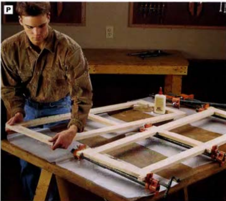
PHOTO P: Make dowel joints at all the rail/stile joints on each cabinet door, then glue the joints and assemble the door frames. Position a bar or pipe clamp beneath each rail location and use clamp pads to protect the wood.
