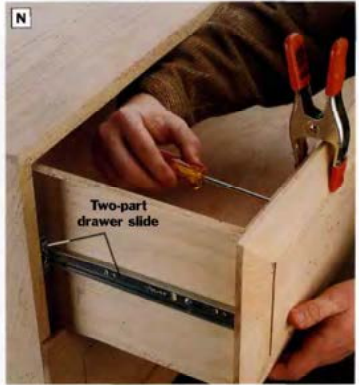
PHOTO N: Attach the drawer fronts to the drawers with screws driven through the front, inside face of the drawer box and into the back face of the raised-panel drawer front. Hang the drawer boxes first so the drawer fronts will be perfectly positioned.
