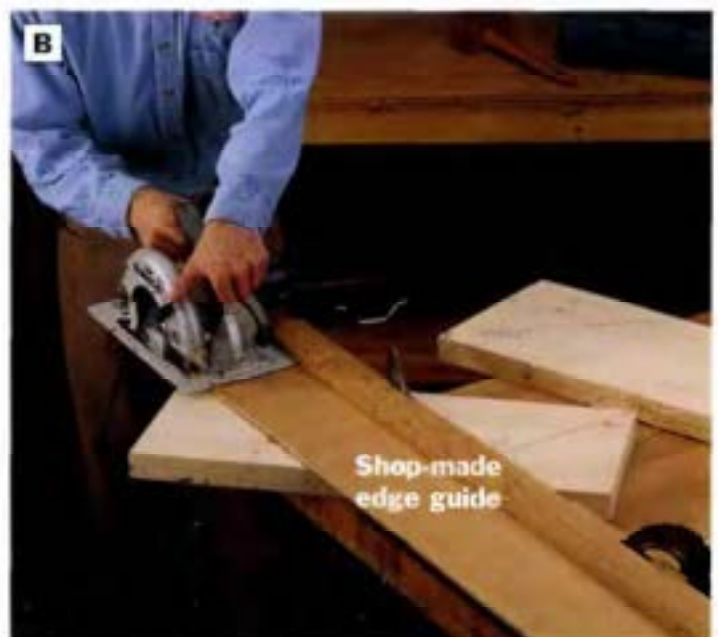
PHOTO B: Gang-cut the carcasse top and bottom panels to size, then gang-cut the fixed shelves. Use an edge guide clamped to the workpiece and your workbench to ensure straight cuts.
