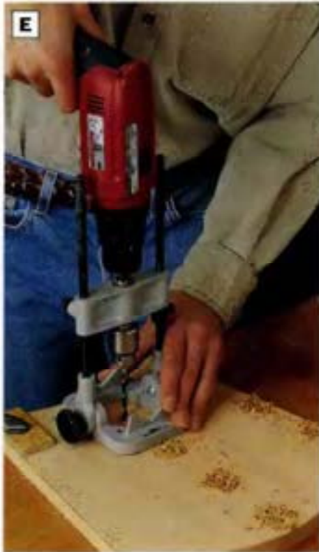
PHOTO E: Drill 1/2-in.-deep dowel holes at the dowel hole centers you marked on each of the two sides with the hardboard template. Use a drill guide to ensure straight holes.
