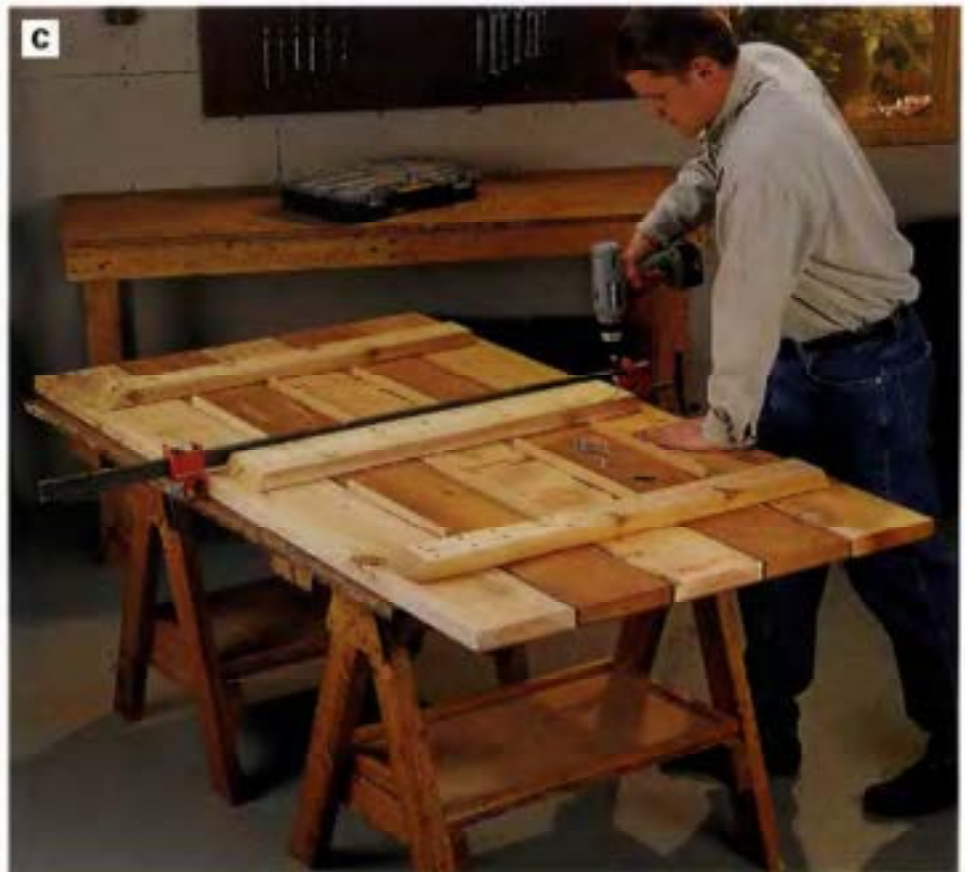
PHOTO C: Mark locations for the three table stretchers on the bottom of the tabletop, then fasten the stretchers to the table slats with 2½-in. galvanized deck screws. Set ¼-in. spacers between the slats before you fasten the stretchers to keep the slats held evenly apart.
